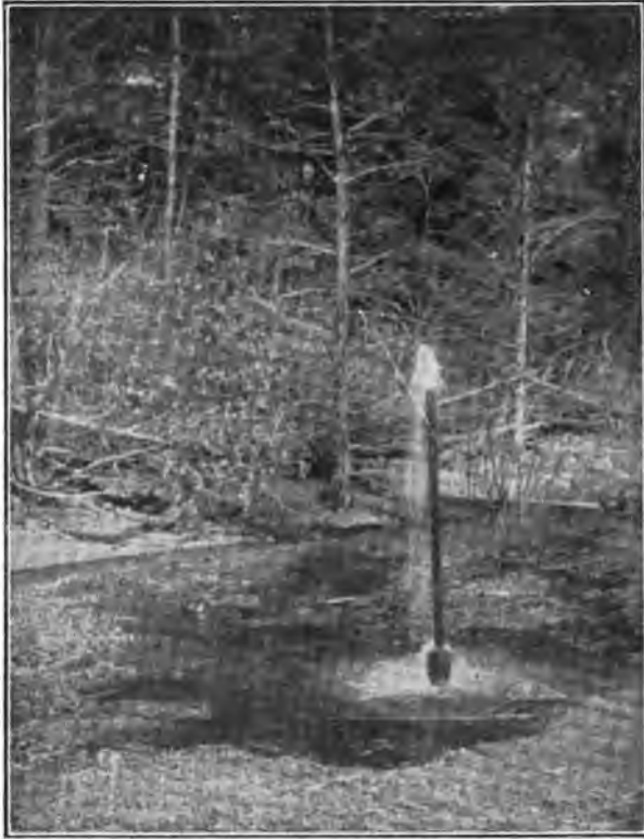
PLATE 79.—Spouting Diamond-drill Hole over Tunnel. This hole ceased to flow when tunnel was driven below. Flow renewed when lining was grouted.
